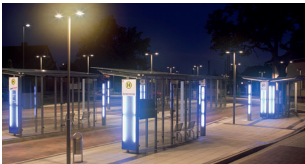
Photos 62 and 63: The light is required to enable passengers to identify stopping areas and bays and to clearly distinguish ground, steps and floor when entering and exiting vehicles.
